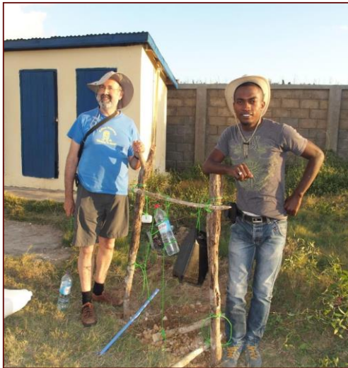
Constructing a Tippy Tap—a simple hygienic construction for hand washing with running water.
